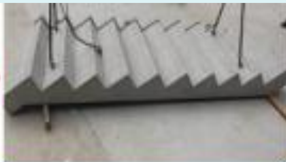
楼梯构件起吊
